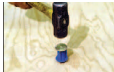
Wood-Form Insert Installation Sequence
